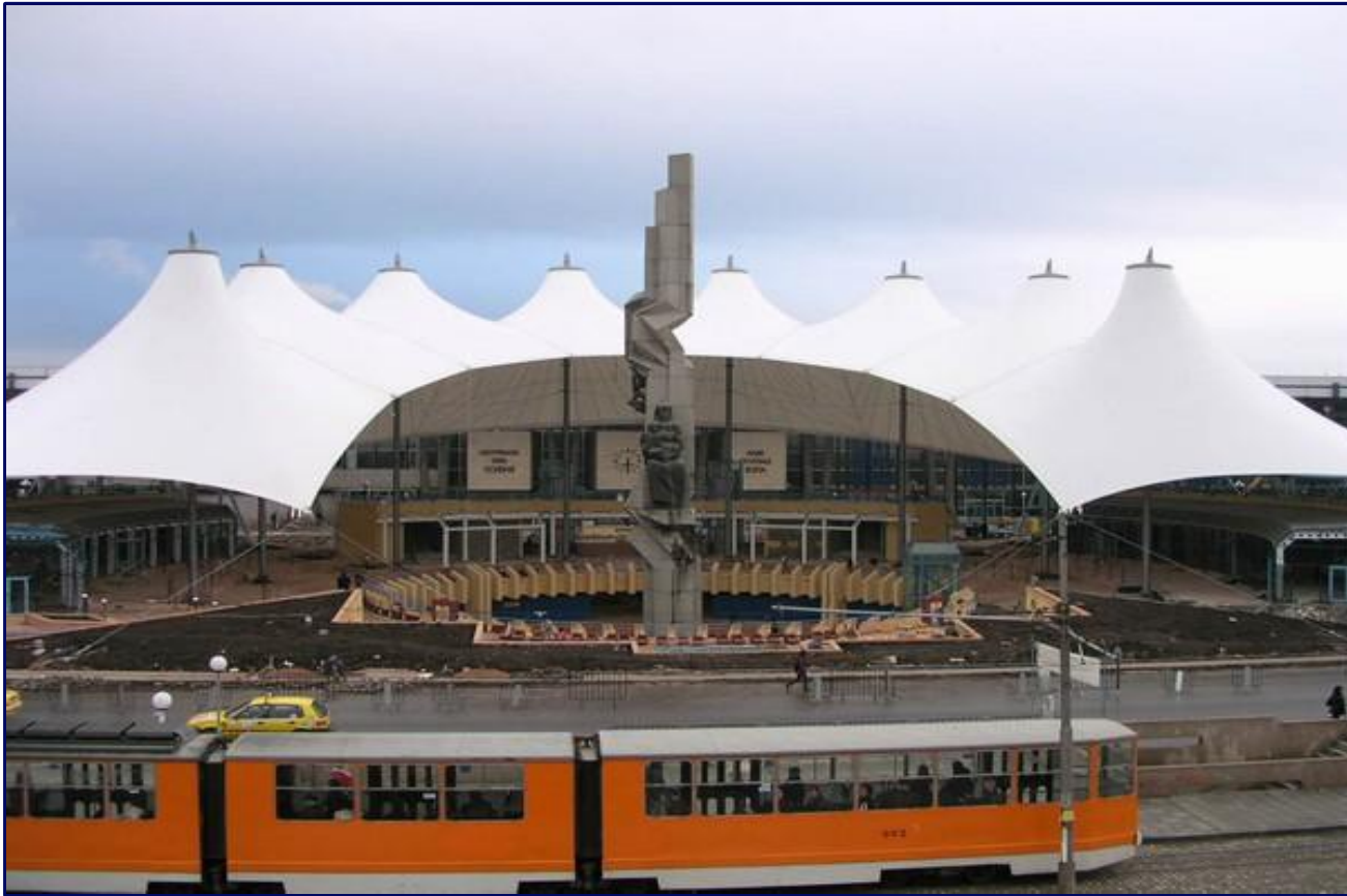
Project: Central Station with pipe supports (Sofia)
